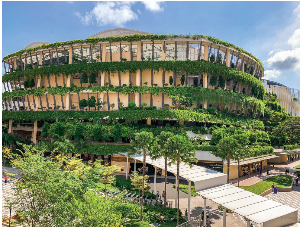
A variety of greenery – trees, shrubs and creepers, envelopes the mass of the building, mitigating its visual impact on the massing. They serve as natural screens for the indoor areas by reducing heat gain.
