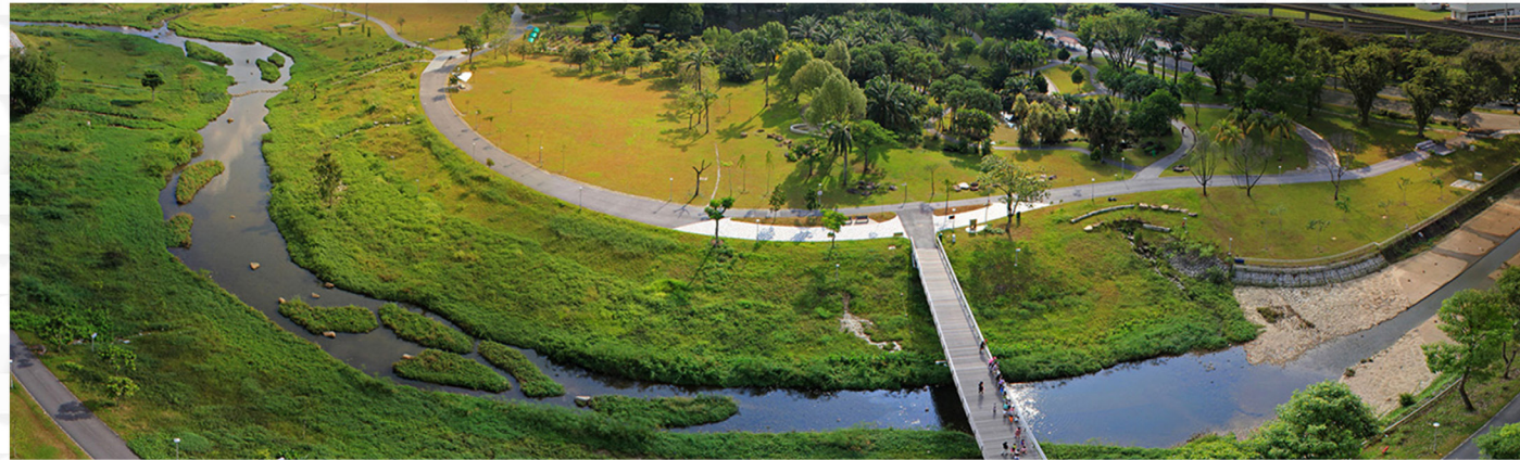
Kallang River transformation at Bishan- Ang Mo Kio Park Image courtesy Ramboll, Singapore
