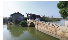
Shangxianhe Wetland Park Area: 210ha Design/Completion: 2007-2009/2011 Award: • Second prize of 2nd Landscape Planning and Design Awards, Chinese Society of Landscape Architecture(CHSLA), 2013
